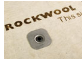
Installed plastic tube and washer
