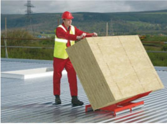
Use of the Rockwool Rock Roller trolley allows fast and easy movement of boards across the roof decking
