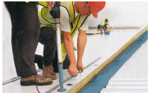
Typical installation of a single ply membrane over Hardrock Dual Density roofing boards.
