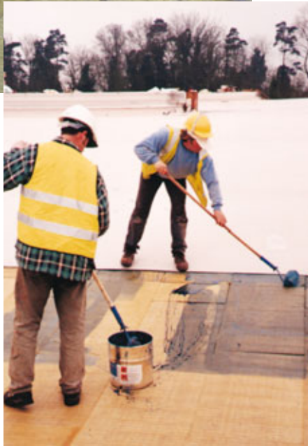
Application of adhesive to Hardrock Dual Density SPA.
