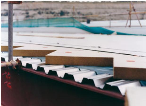
Hardrock Dual Density roofing boards applied below mechanically fastened single ply membrane.
