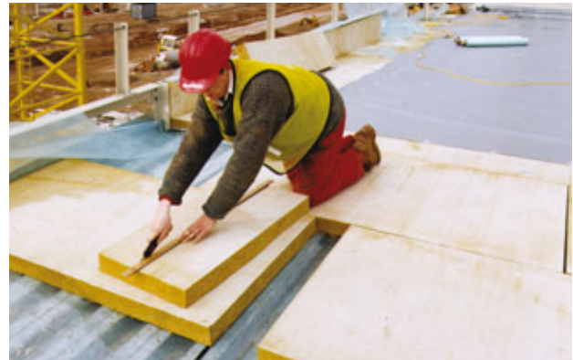
Hardrock Dual Density can be easily cut and shaped on site where required.
