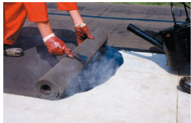
Typical pour and roll application over Hardrock Dual Density Tissue faced roofing boards
