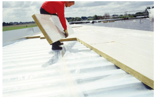
Typical installation of mechanically fastened Hardrock Dual Density (Tissue faced) roofing board, on a profiled steel deck, incorporating a single ply membrane.
