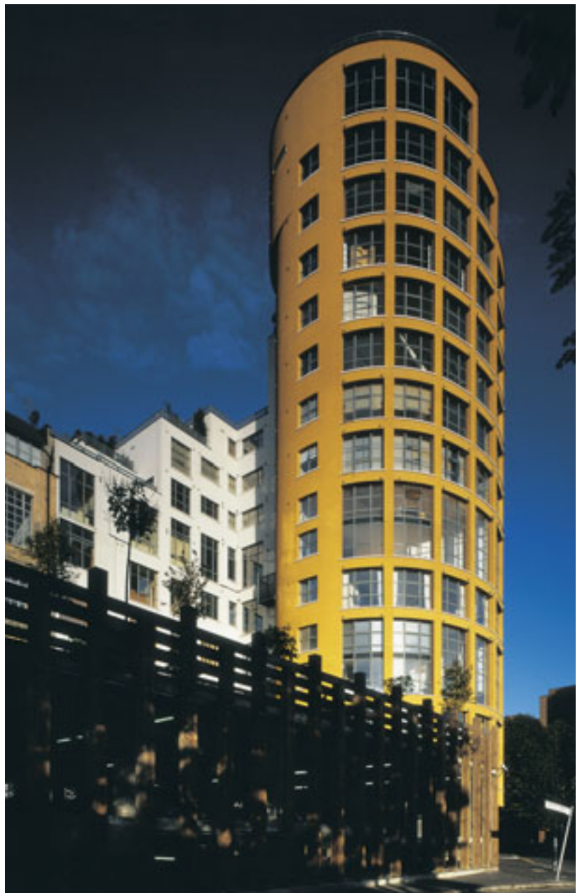
Bankside Lofts, London SE1 Architects: CZWG
