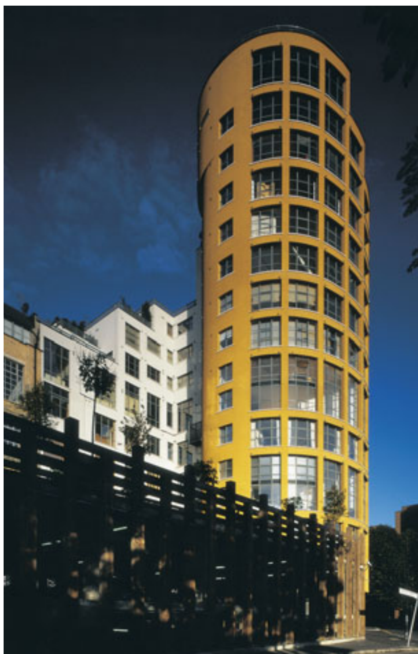
Bankside Lofts, London SE1 Architects: CZWG
