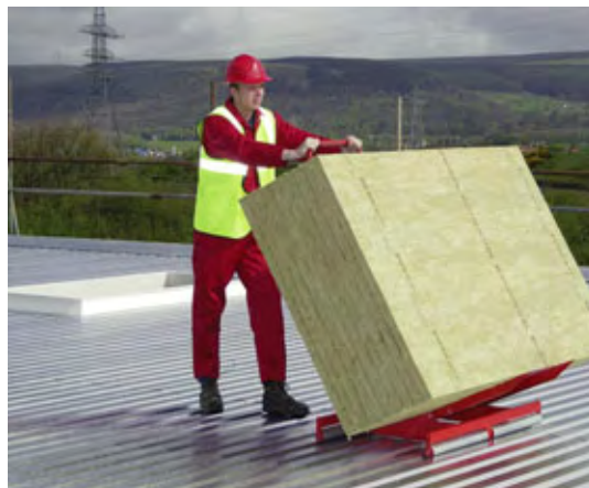
Use of the Rockwool Rock Roller trolley allows fast and easy movement of boards across the roof decking
