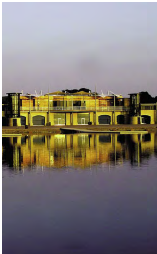
Eton boat house. DuoRock (Plain) roofing board. 1,200m 2
