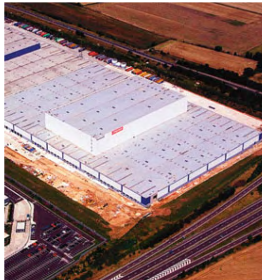
IKEA Distribution centre, Doncaster. DuoRock (Plain) roofing board. 80,000m 2
