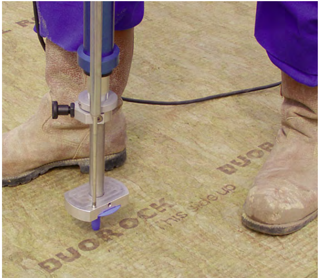
Application of a plastic tube fastener
