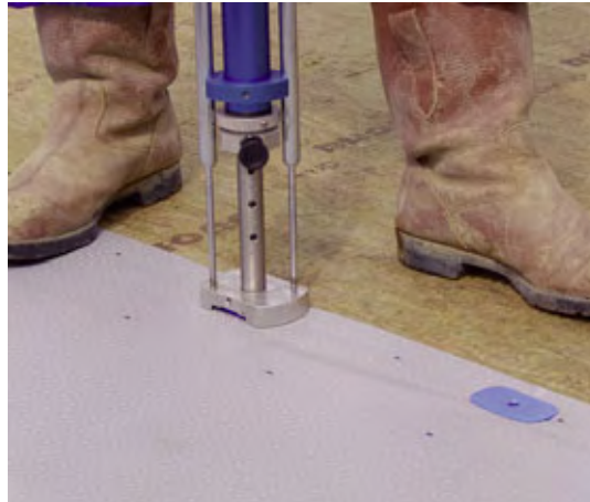
Typical application of a single ply membrane over DuoRock (Plain) roofing boards
